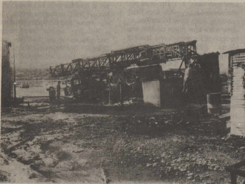
The aftermath of the fire. The pulling unit & several tanks were destroyed. Damage estimates could go as high as $1 million.
