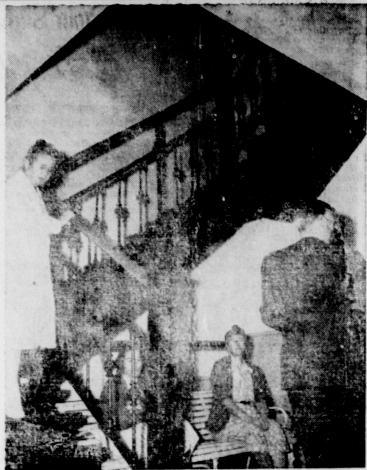
IRON STAIRS IN ABILENE HOSPITAL — This ancient iron stairway at the Abilene State Hospital has caused many falls—not only by the epileptic patients in the hospital, but by the nurses as well. Several patients in the last dozen years have fallen on those stairs and been killed. Injuries occur nearly every week. Notice how cautiously the nurse in the picture is moving from step to step. Abilene State Hospital was one of the several hospitals at which newspapermen of the state recently inspected conditions.
