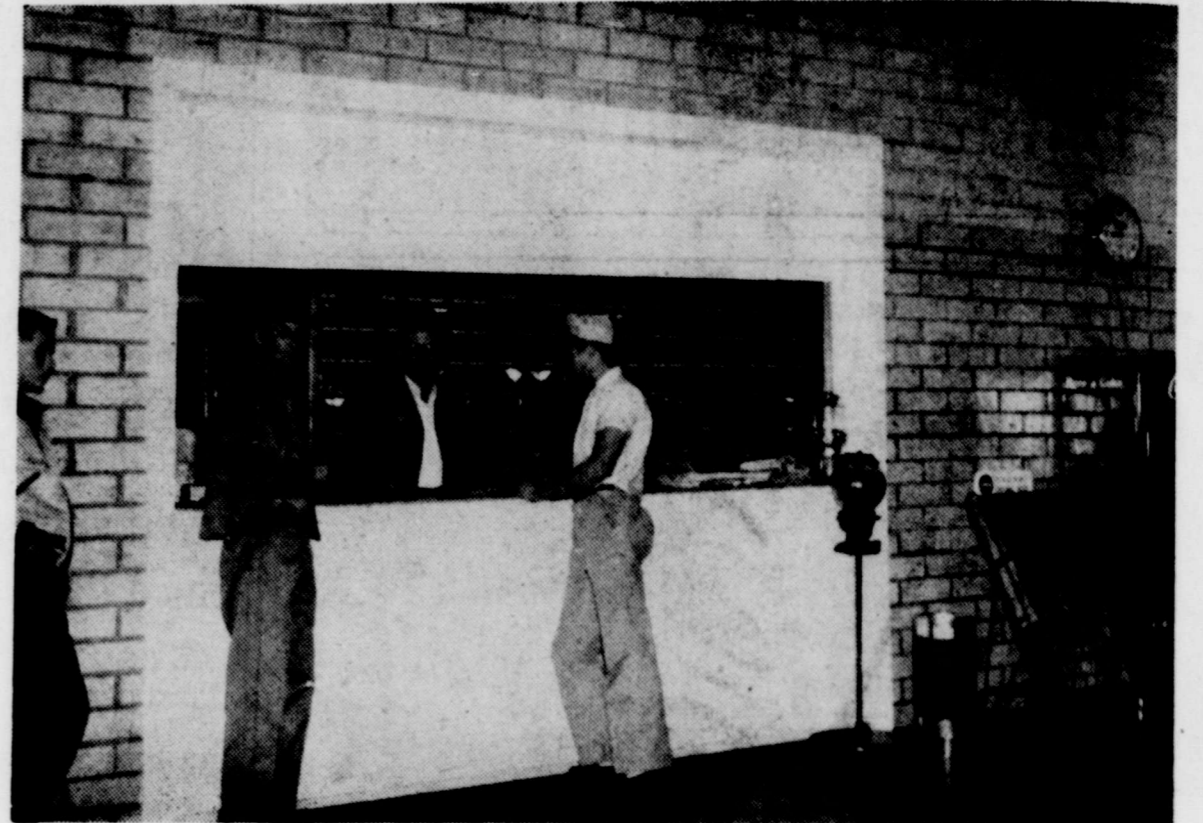
Window Opening From Parts Department Into Shop
