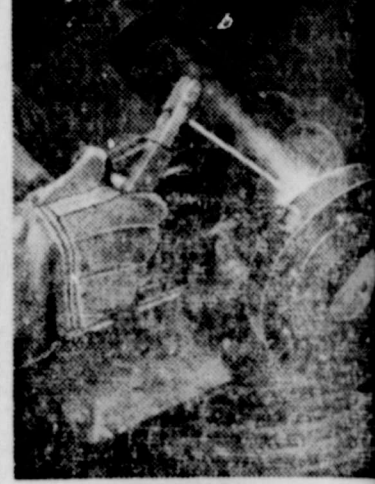
THEY WELD PIPE
