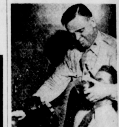
BABY LUNG . . . Use of portable automatic baby lung developed by army air forces is demonstrated by Capt. Hurley L. Motley. The light-weight lung, it is believed, will replace the cumbersome iron lung in cases of infantile paralysis.
