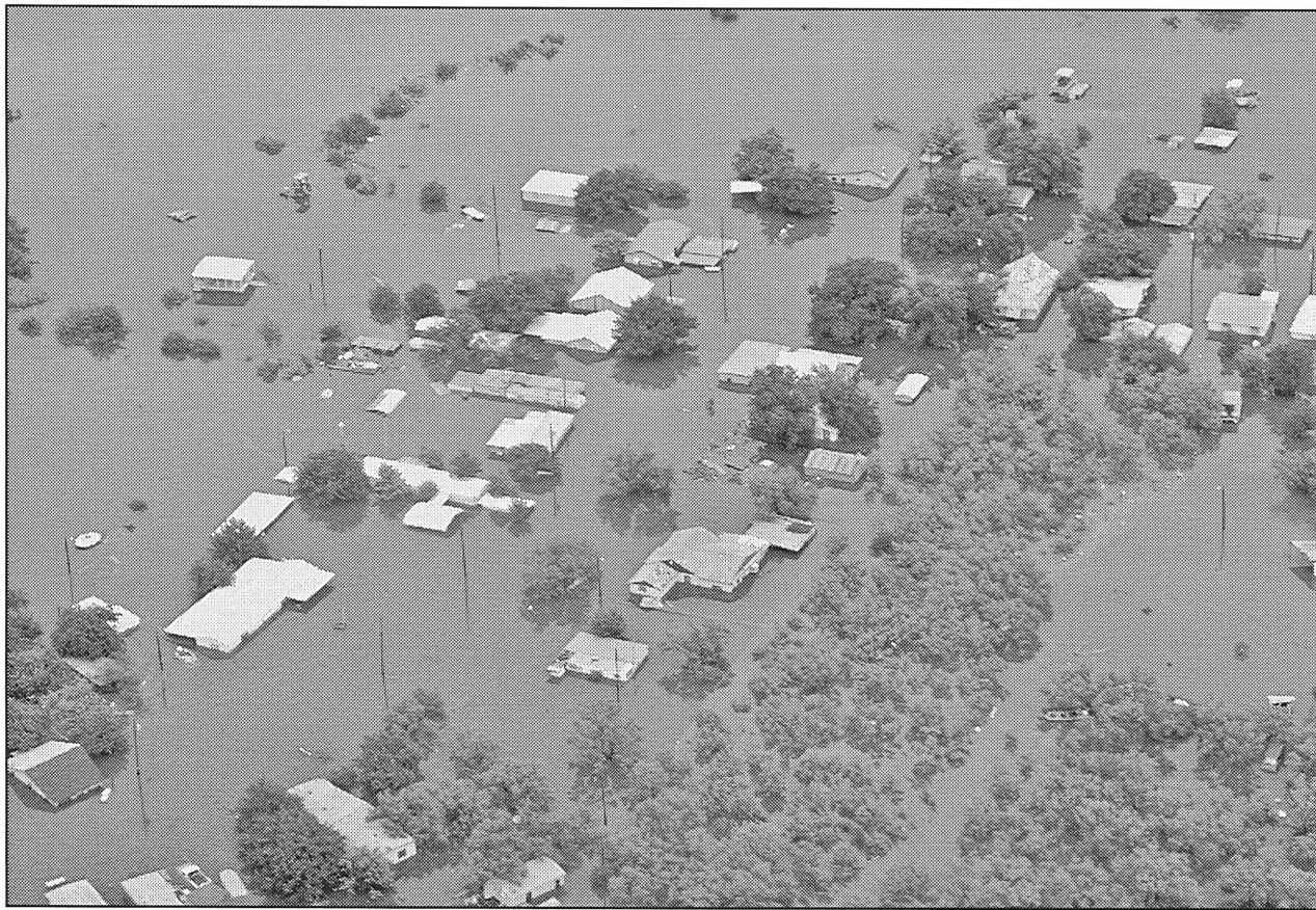
A BIRD'S-EYE VIEW —An overhead shot of Jeffcoat's Camp taken from the Texas Department of Public Safety helicopter making a survey of flood damage to the Lake Stamford area, shows some of
