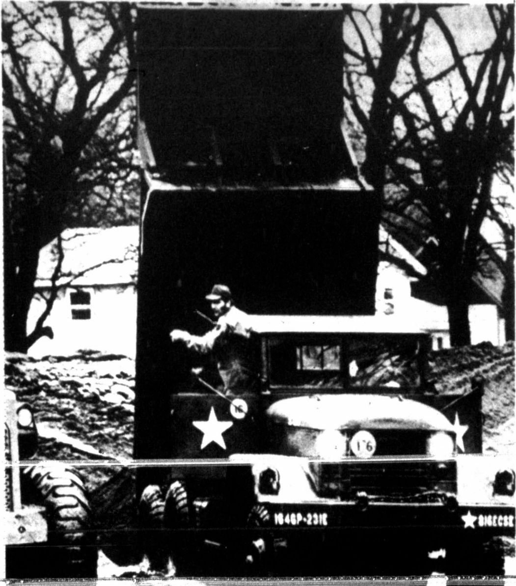
A NORTH DAKOTA National Guardsman dumps a load of clay on the backup dike in the Riverside area of Grand Forks Tuesday as efforts continued to keep the dike holding back the flood waters of the Red River, which already claimed the home in background and several others after the main dike broke Monday.
