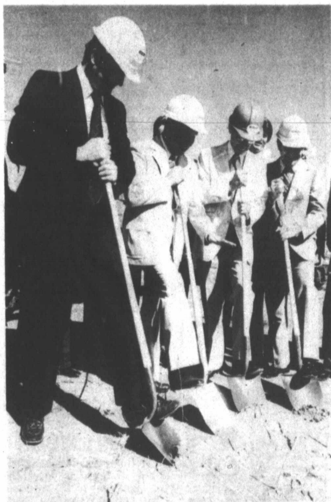
GROUNDBREAKING for the 200,000 square-foot Pampa Mall began Aug. 1 by Ainbinder Associates, a Houston firm that is building the mall. The mall is expected to be completed in the fall of 1979.
