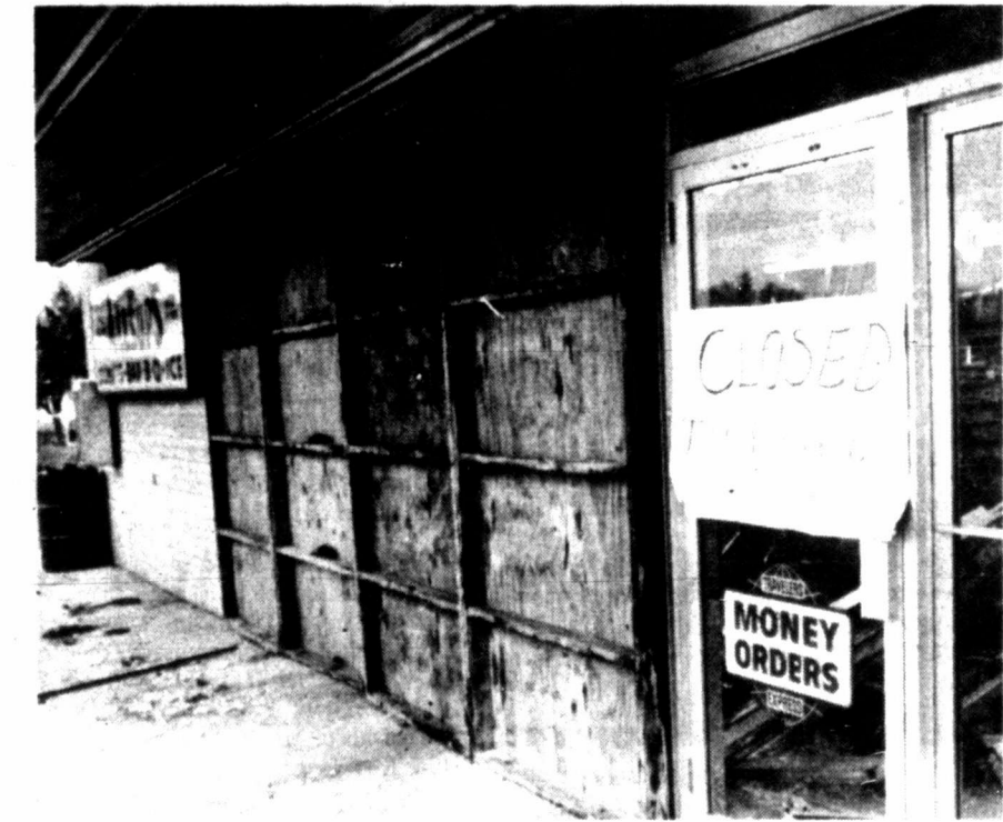
ALLSUP'S CONVENIENT STORE , 500 E. Foster, was suddenly remodeled at 1 a.m. Sunday when a male drove a pickup truck through the front of the store, destroying the counter and causing damage estimated at $5,000-10,000. The driver fled the scene in the truck, described by witnesses as a blue Ford. (Pampa News photo by John Price)
