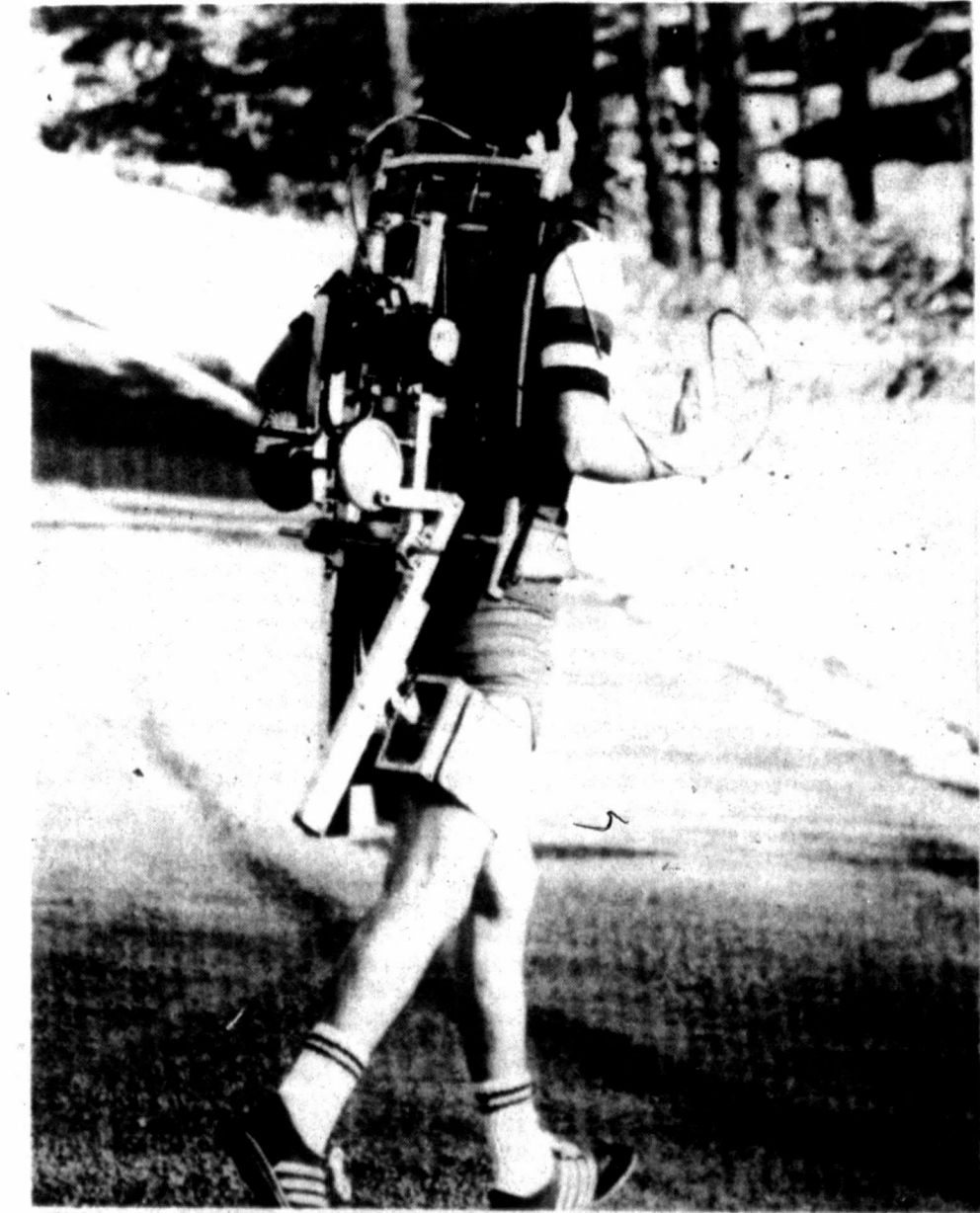
BURT M. SHULMAN of Hyde Park, N.Y., demonstrates the jogging machine that he invented. The machine propels the runner at variable speeds up to 25 mph when strapped to the back like a backpack. (AP Laserphoto)
