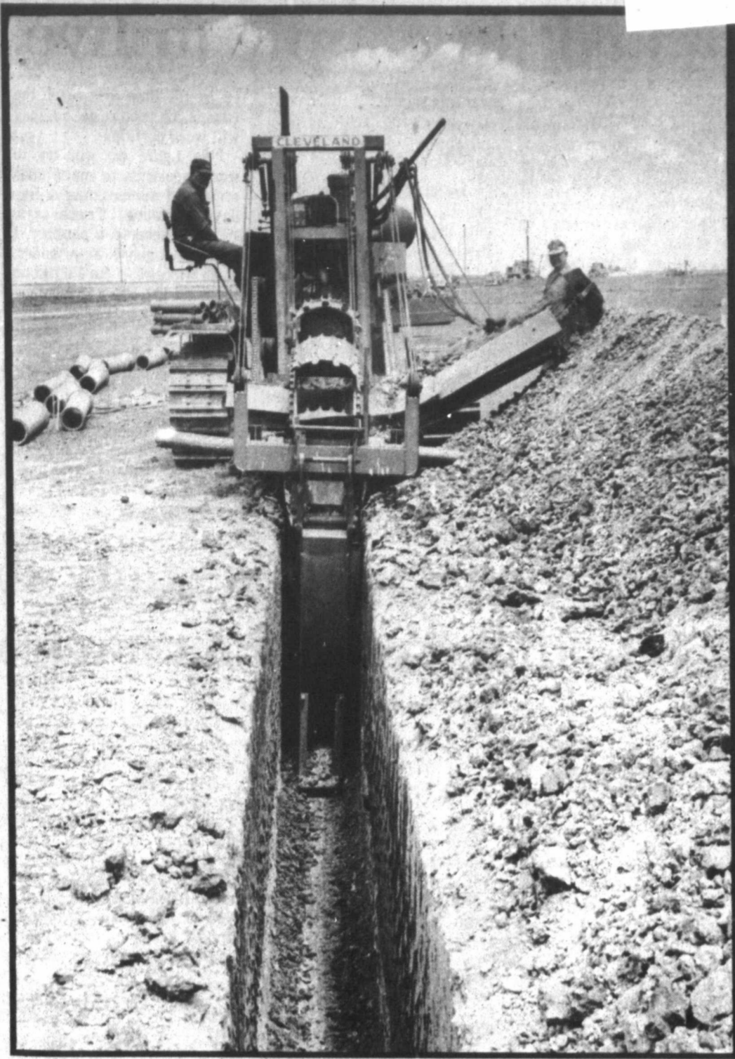
Digging is Progress
