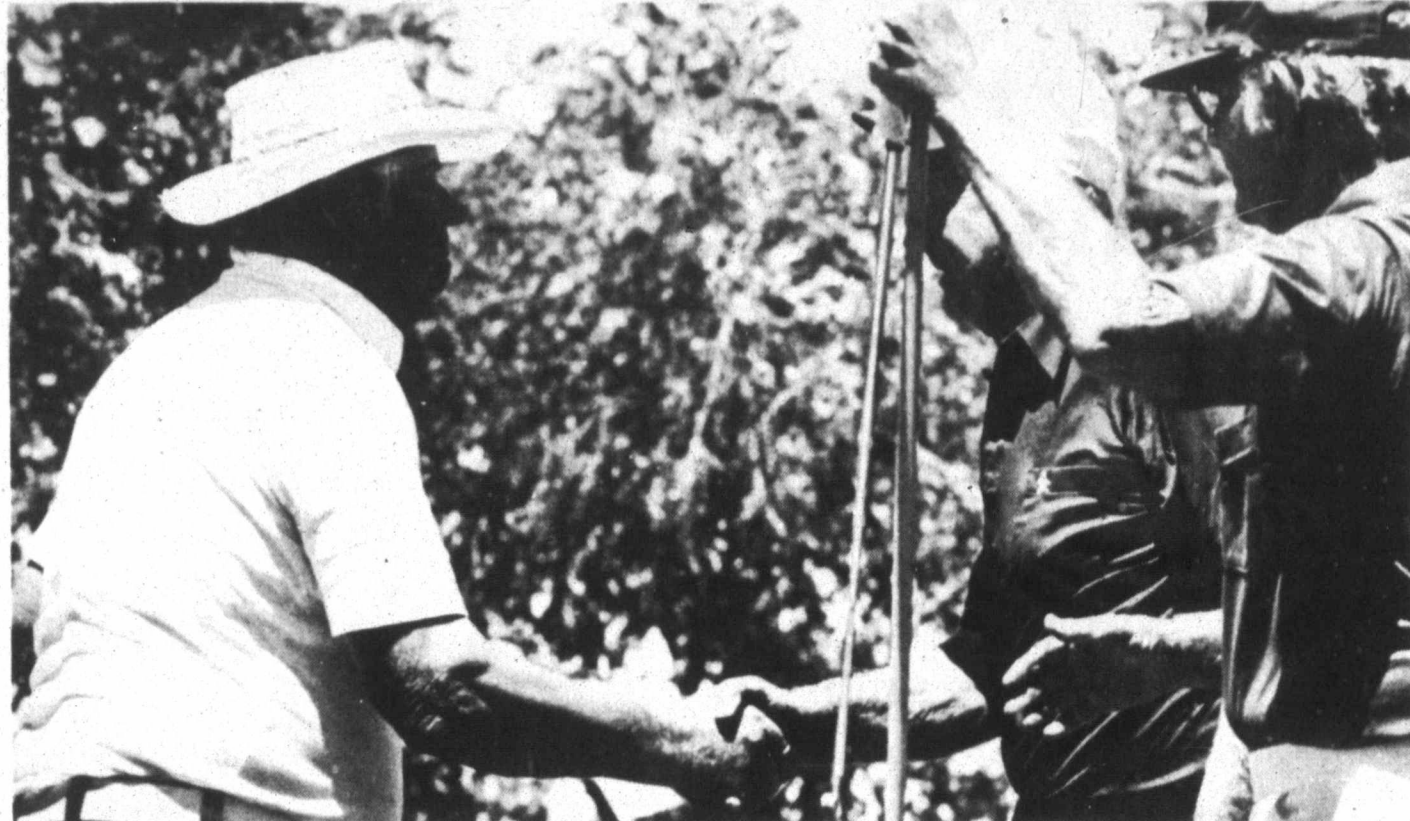
Job well done
