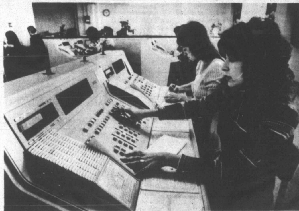
Southwestern Bell's introduction of Zero-Plus Dialing in Pampa means that operators in West Texas cities will now be handling Pampa operator-assisted calls from new consoles like these.
