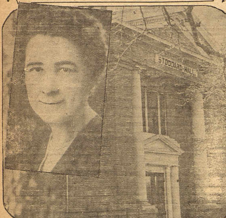
President L. H. Hubbard, pick in hand, begins wrecking of Stoddard Hall, first state dormitory at Texas State College for Women (CIA), which will be replaced through PWA grants by a modern four-story, fire-proof building. The lower picture shows old Stoddard in all the glory of former days, and (inset) Miss Jessie H. Humphries, first director, now associate dean of the college.
