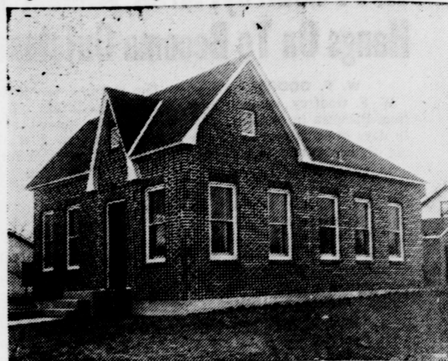
PICTURE of Southwestern Bell Telephone before present additions were made
