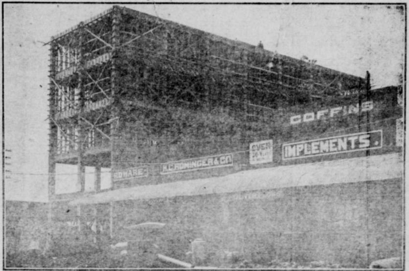
The above picture was taken some few days ago of the new building for the Cisco Banking Company. As you will notice this building is five stories high, and the walls are now being constructed. This will be of dark brick with white stone as bases and outlines. This will be a bank building on first floor and offices on the other floors and will cost \$100,000.00.
