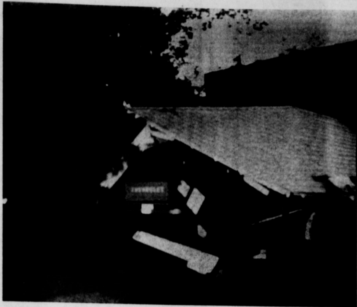
STORM DAMAGE—This wash house at the Vernon Chew Station was twisted and torn in last Thursday's wind storm. Barely visible under the structure is a pickup belonging to Chew, and a diesel pump. A large tree to the left of the house was also twisted.
