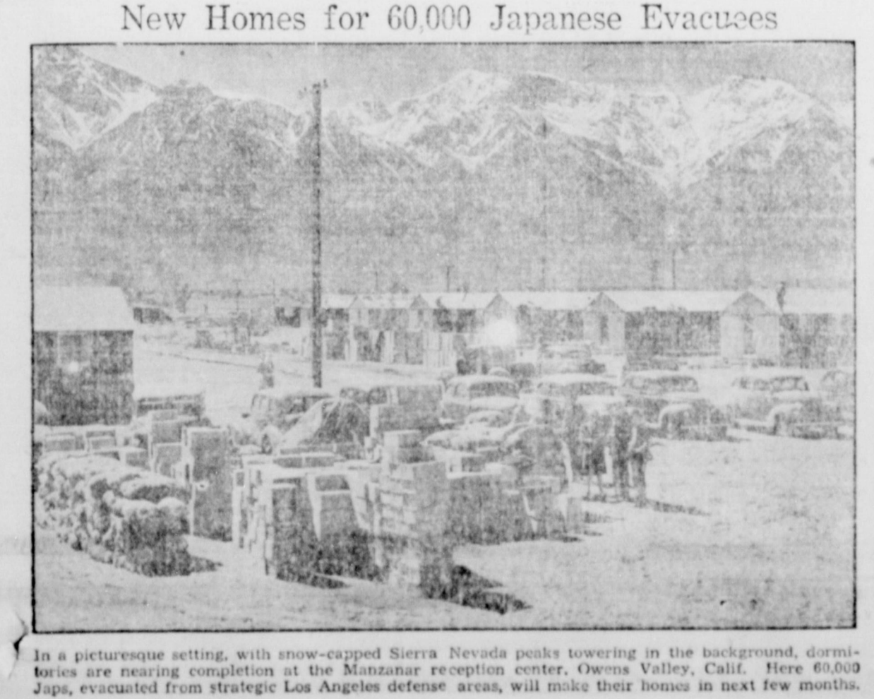
In a picturesque setting, with snow-capped Sierra Nevada peaks towering in the background, dormitories are nearing completion at the Manzanar reception center, Owens Valley, Calif. Here 60,000 Japs, evacuated from strategic Los Angeles defense areas, will make their homes in next few months.
