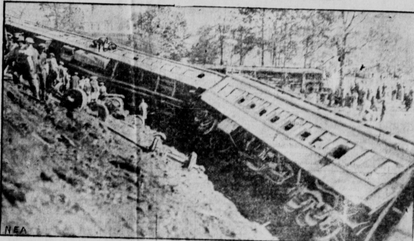
When the "Sunnyland," crack flyer of the Frisco railroad, jumped the rails and plunged down a 40-foot embankment near Victoria, Miss., 19 persons were killed and more than 60 injured. This remarkable picture shows a group of rescue workers on the second pullmen trying to pull one of the wounded passengers out through a window. The train was traveling about 55 miles an hour at the time and this speed caused one car to be hurled nearly 75 yards from the track. The under framework of this car can be seen in the adjoining picture.
