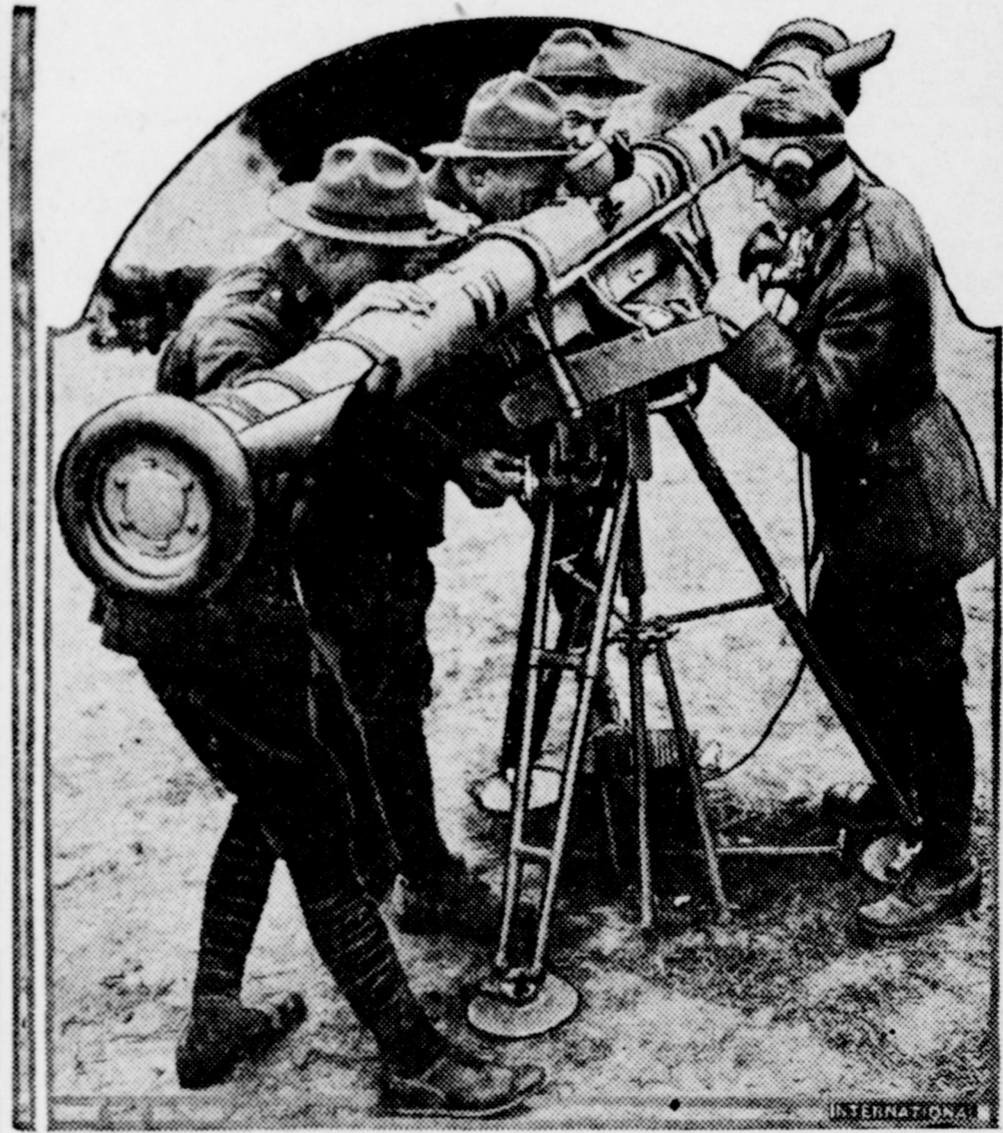
Officers looking at the belemeter, the newest device aiding anti-aircraft guns to locate the target and helping to obtain the slant range for the guns. This and other new devices were demonstrated at the seventh annual meeting of the Army Ordnance association, and other organizations interested in ordnance and defense.
