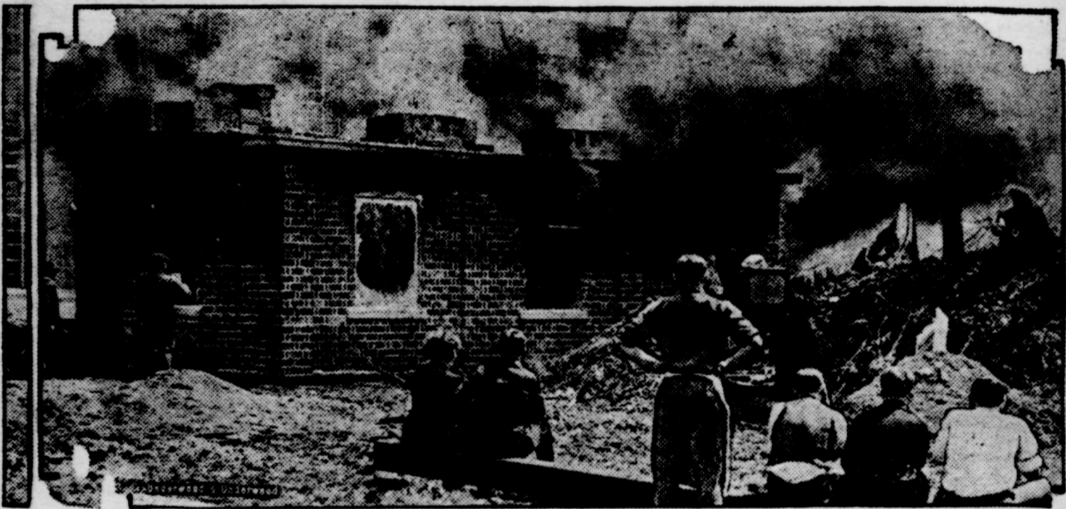
Unusual, is it not, to see a group of husky men stand back and watch a house burn? But it was only a test made at the bureau of standards in Washington with a so-called fireproof building filled with safes, filing cabinets and some combustible material, to determine just how much fire and heat they would stand.
