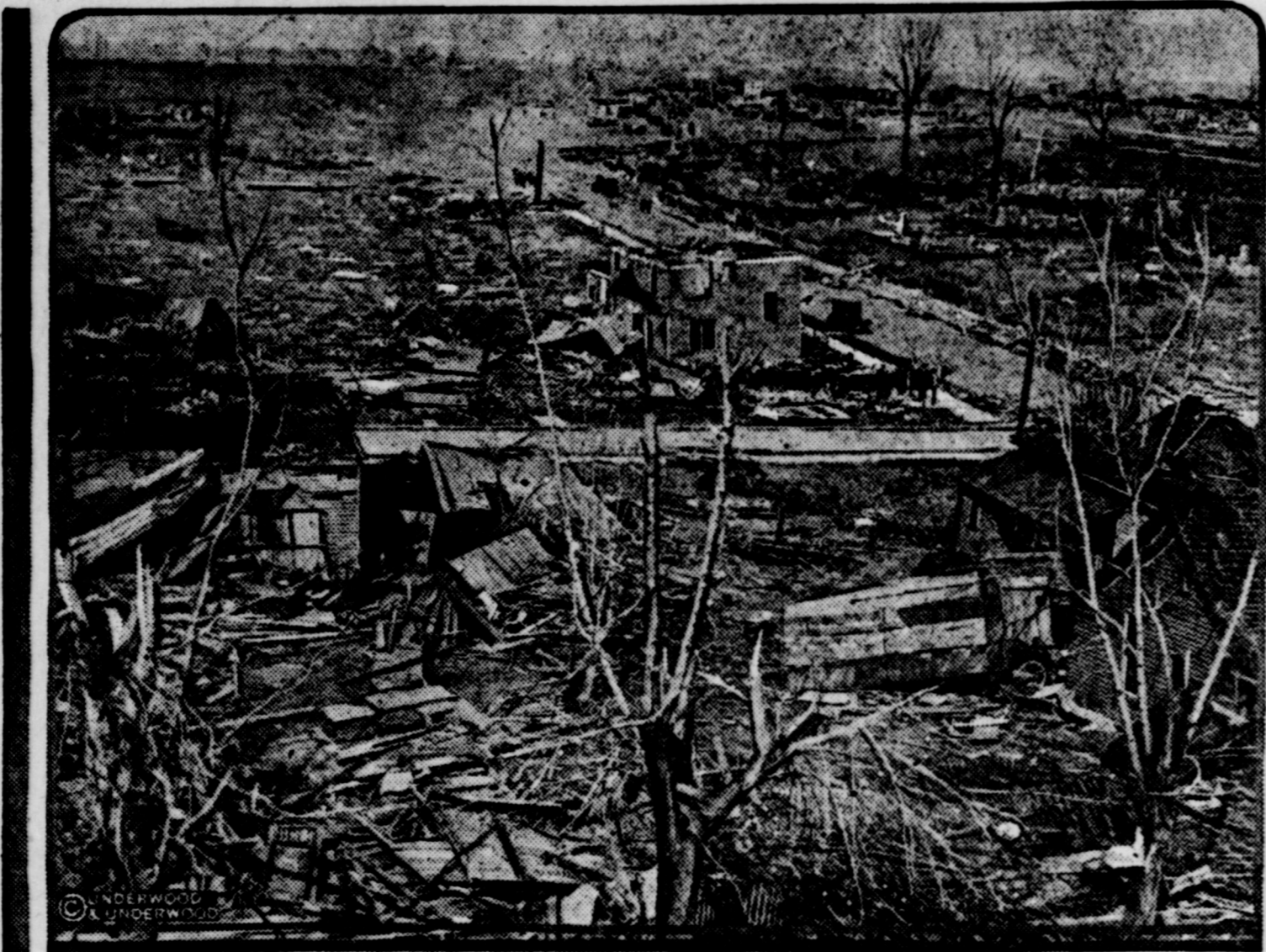
This is a panoramic view of the devastation caused throughout southern Illinois by the recent hurricane in which hundreds of lives were lost, many hundreds of people seriously injured, and millions of dollars' worth of damage resulted.
