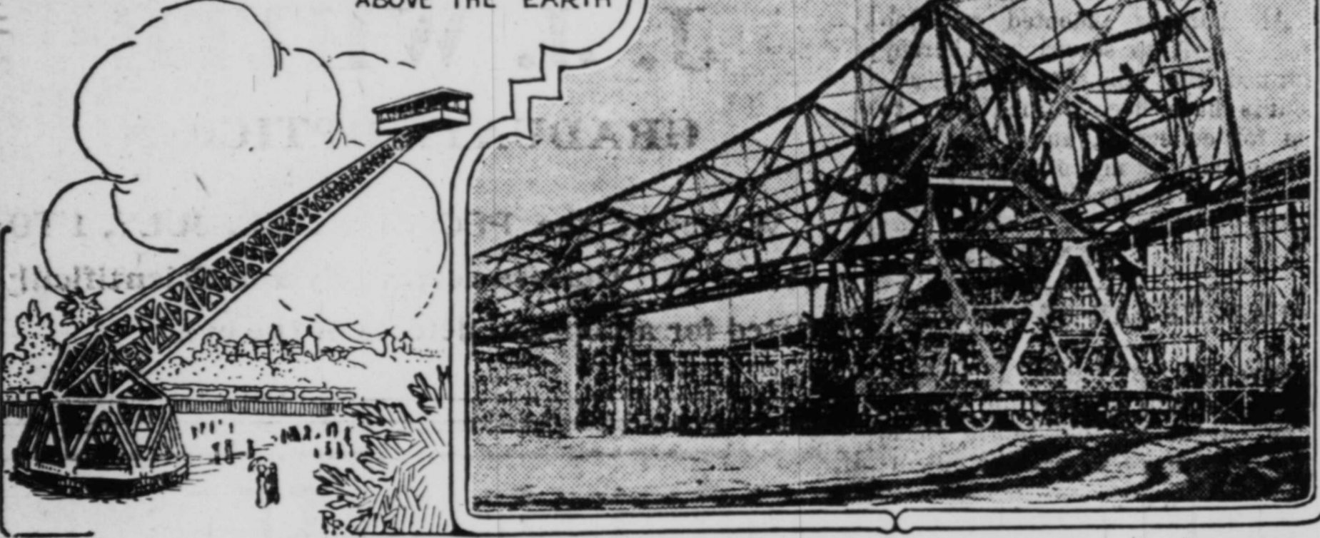
THE GIANT FRAME OF THE AEROSCOPE AS IT APPEARED UNDER CONSTRUCTION
