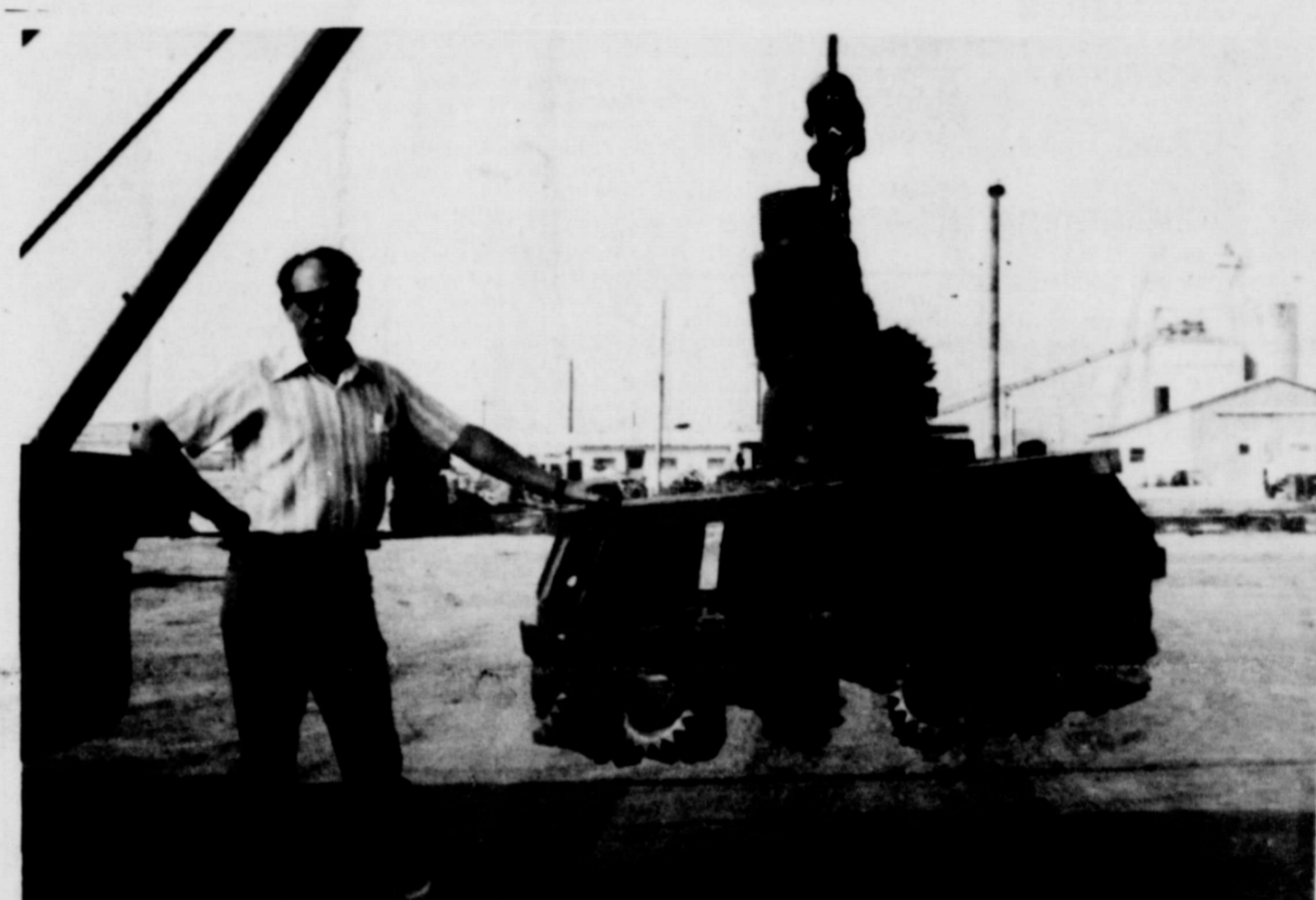
Roy Bulls is pictured above with one of the large bits used in the "raised bit" drilling process, used by Spearman's Baker-Taylor Unit.
