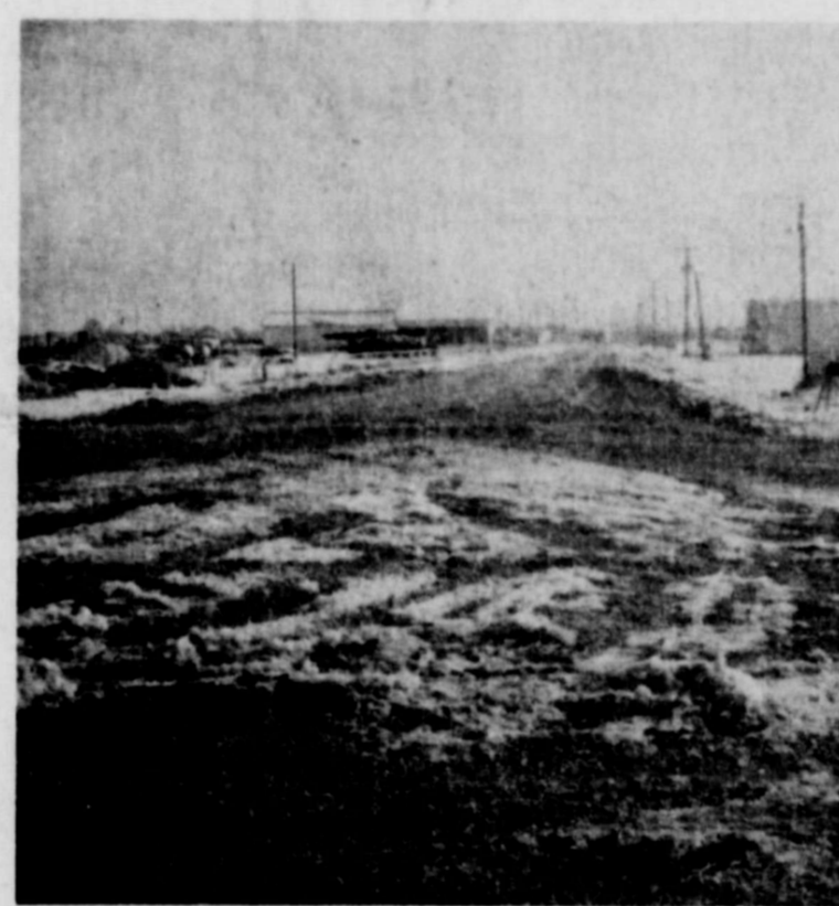
The County Commissioners court agreed to work over this section of 7th street for the City of Spearman and workers completed the job last week before the snow fell. The extension of 7th street is located from highway 207 west to the paved county road which runs N & S in front of the Spearman animal clinic. County funds, equipment and labor were furnished and the road received a nine-inch topping of concrete to put this much-used road up in top shape and all-weather proof. "Kudos" to the commissioners for this job.
