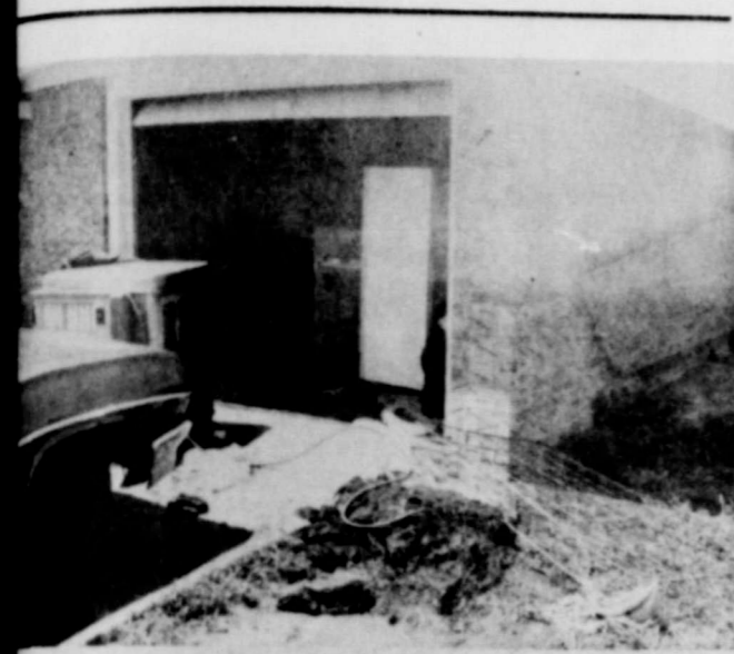
THE FIRE ALARM which sounded at 1:30 p. m. Monday turned out to be only a mattress on fire in the garage at the Reyes Castenada residence, 712 Cotter Drive.
