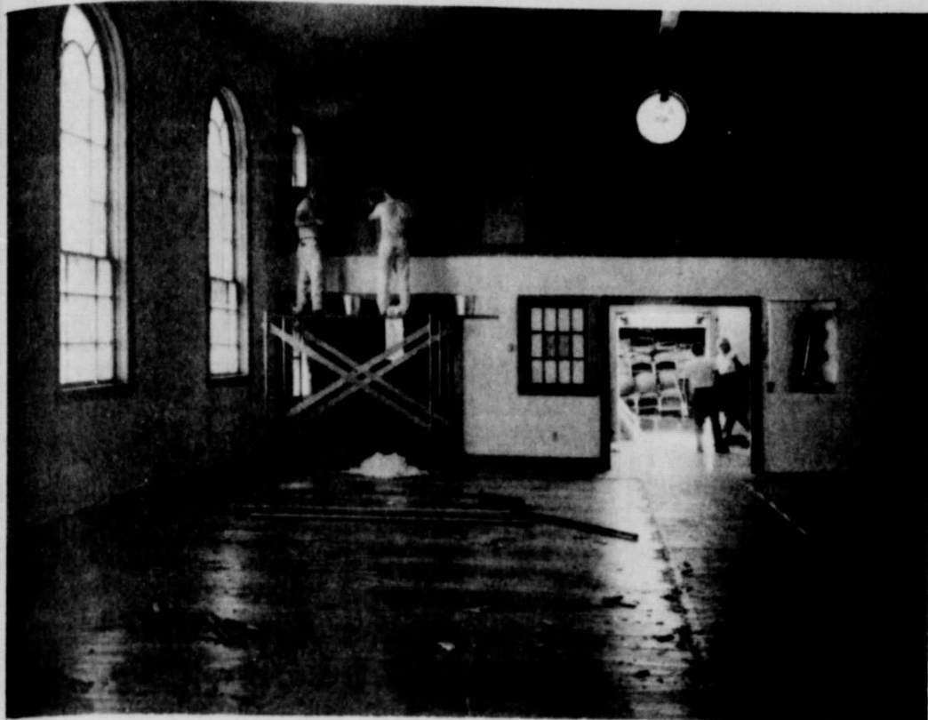
REDECORATING JOB UNDERWAY---This is the way the Sanctuary of the First Baptist Church looked Tuesday morning. Workmen had completely gutted the building, beginning an extensive redecorating job which is supposed to be completed within the next 5 to 6 weeks. The sanctuary will be out of use only 4 Sundays.
