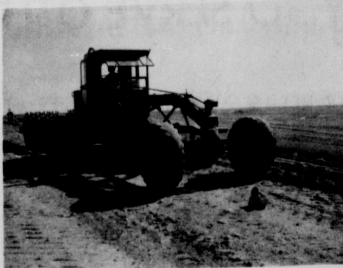
some grader work done...
