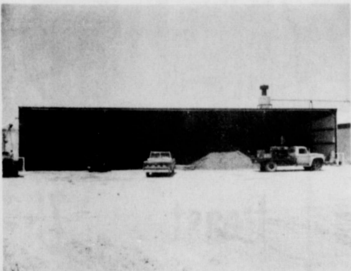
FEED PROCESSING PLANT AND STORAGE AREA.
