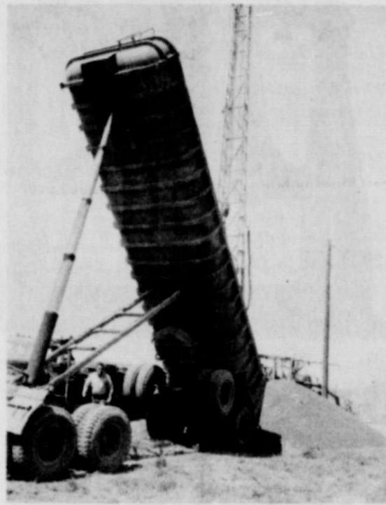
Gravel for the new water well at Hansford Feedyard is being unloaded above.
