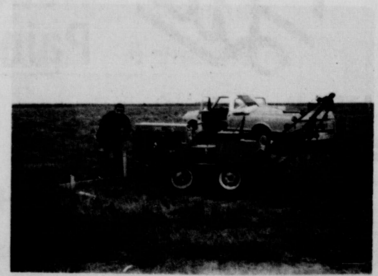
Maxey Baker stakes out the feed mill foundation.
