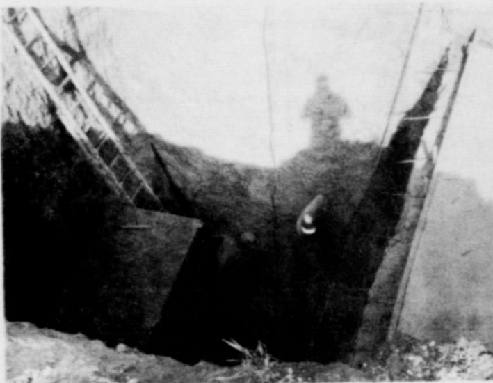
Ground work for feed mill
