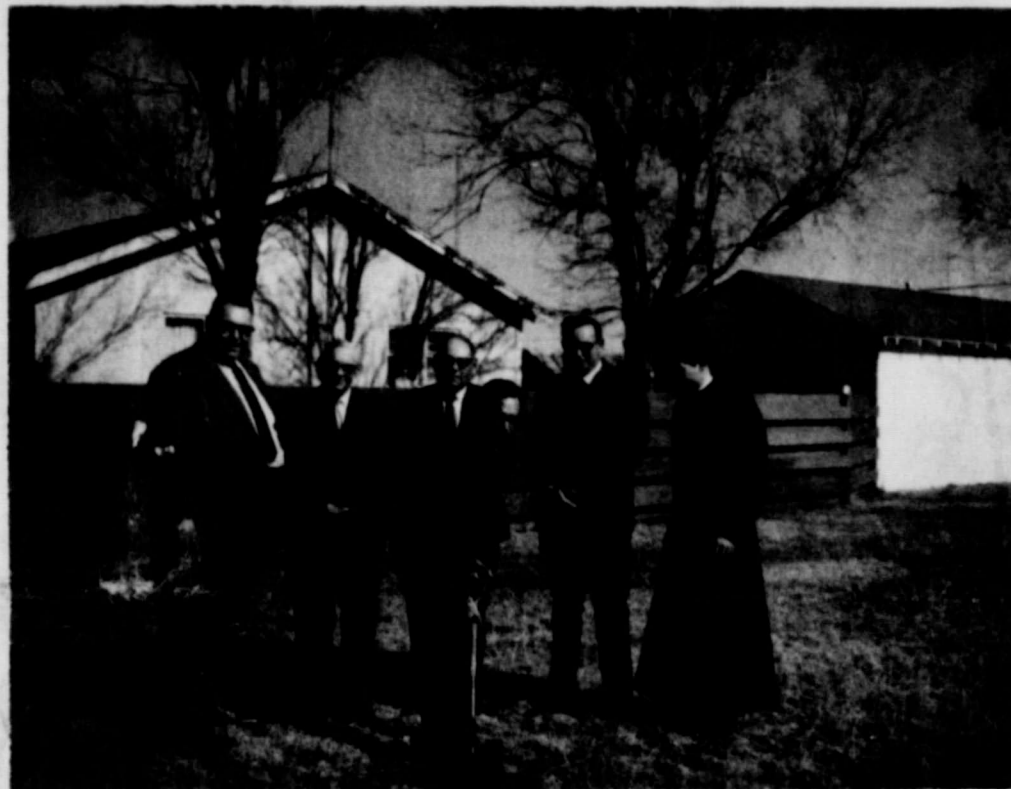
GROUND-BREAKING CEREMONIES--held recently for the new Sacred Heart Fellowship Hall at the Catholic church, shows Carlos Lopez spading the first shovel of dirt. Building committee members pictured with him are, L to R: Dr. R. L. Kleeberger, Gus Renner, Clarence Renner, Jerry Morris and Father Donald P. Rusch, pastor.
