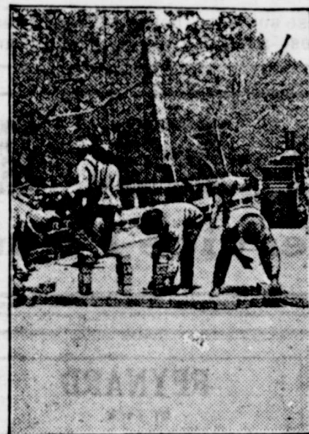
Laying Vitrified Blocks.
