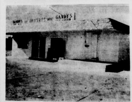
Workmen were putting the finishing touches on a new bit of "head dress" this week at the Rankin Drive-In Grocery at Grand and Hwy. 67. Featuring the wooden shingles and extended eves, the appearance of the building was much improved as was the shelter during wet weather. Pete Brown was in charge of the job.
