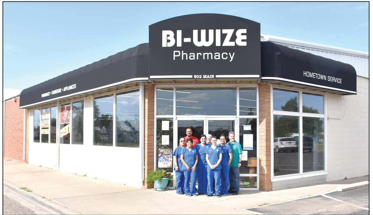
A new store front awning/sign was installed last week at Bi-Wize. The original sign had taken a beating especially this year with the high winds and multiple hail storms. Bi-Wize employees in the picture include (l-r): Peggy Padilla, Raul Dominguez, Olga Legarreta, Saima Rivera, Debbie Williams, Kayla Alexander, Daisy Delgadillo, and Andy Alexander.
