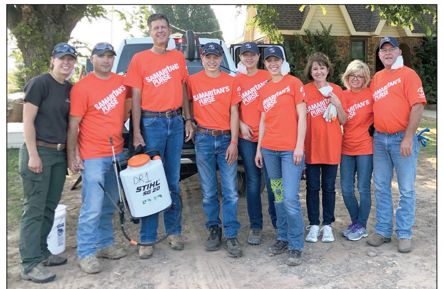
First Baptist Church of Friona sent a work crew last weekend to Fort Gibson, Oklahoma to help clean up and rebuild in the aftermath of recent tornadoes that hit the area. The group worked with the Samaritan's Purse organization which was founded by Franklin Graham, son of the late Billy Graham. Crew members were: (l-r) Debra & Stephen Campbell, Kevin Cooper, Charles Cooper, Faith Cooper, Grace Cooper, Tammy Whiteley, Annette & Kirk Frye, and Pam Hamilton, who took the picture.
