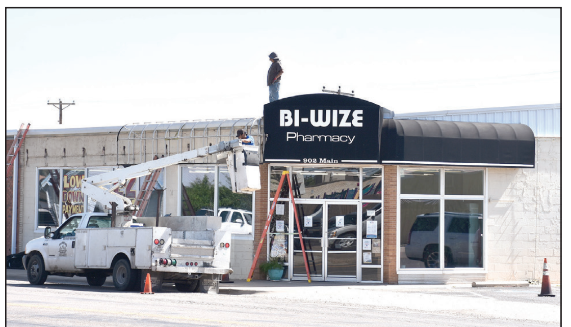
Workers are shown removing the awning/sign from Bi-Wize Pharmacy. After the bomb cyclone event earlier in the year and the repeated hailstorms, the sign was literally hanging on by threads. The awning will be taken to the shop and a new sign will be installed on it.
