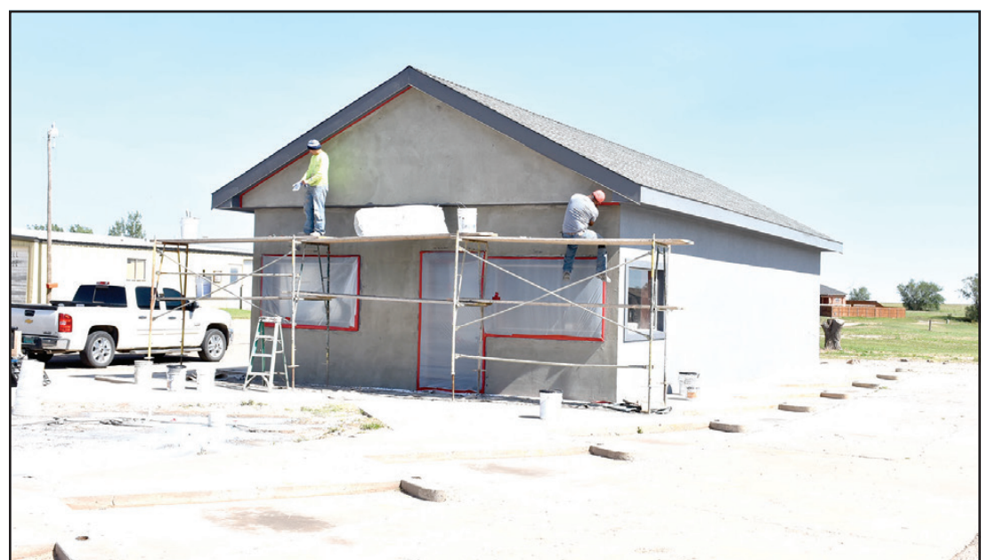
The old Sonic restaurant building is getting a make-over. Improvements include a pitched roof and new stucco exterior. More details later.
