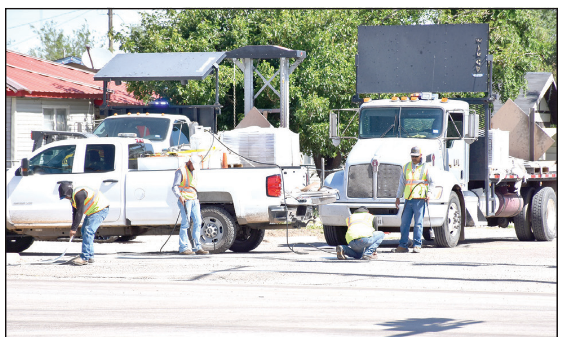
Workers are shown "painting" a new crosswalk at Main and Highway 60.
