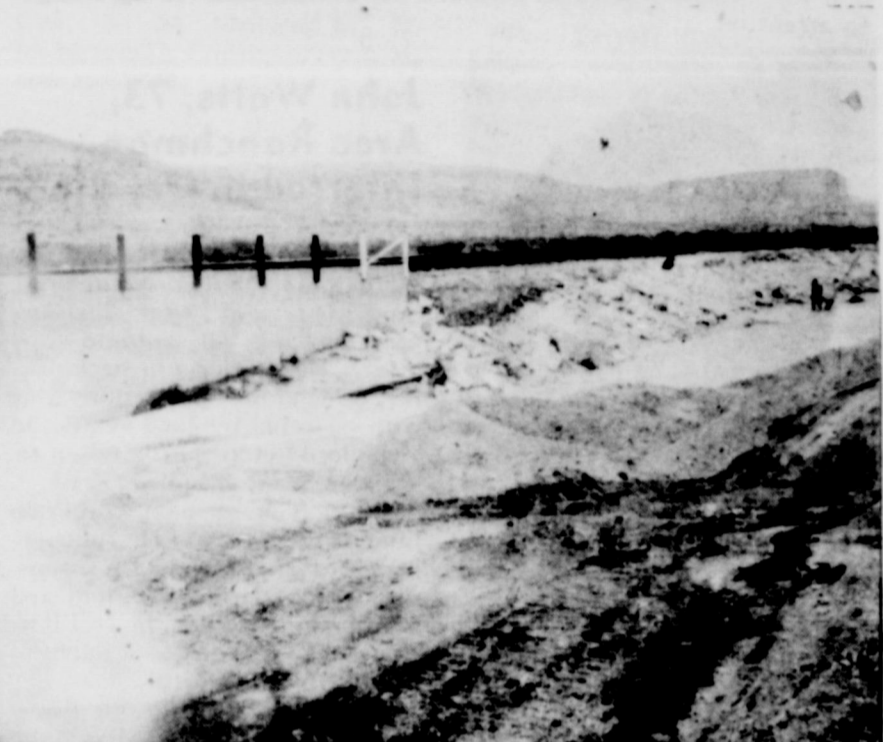
At the top right is a picture taken from where the water came out of Sanderson Canyon showing the beginning of the roadway in the creekbed maintained and used mainly by railroad vehicles. The roadway was cleared for a distance of about 150 yards in the bed of the creek. The pile of dirt and gravel in the center was the result of re-sloping the bank out of the creek.
