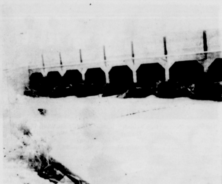
In the picture above the railroad bridge just west of the local gas bulk plants on the west side of Sanderson is shown as it appeared Friday morning following a heavy rain and run-off Wednesday night. The channel of the creek is almost at right angles to the openings under the bridge. A rise in the creek following the collection of brush as shown in the picture might have caused a serious result in forcing the water on to the left which is an extension of Downie St. and parallels the railroad and Oak St.
