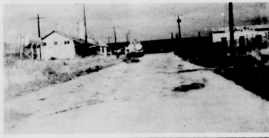
At the top right is a picture taken from where the water came out of Sanderson Canyon showing the beginning of the roadway in the creekbed maintained and used mainly by railroad vehicles. The roadway was cleared for a distance of about 150 yards in the bed of the creek. The pile of dirt and gravel in the center was the result of re-sloping the bank out of the creek.
