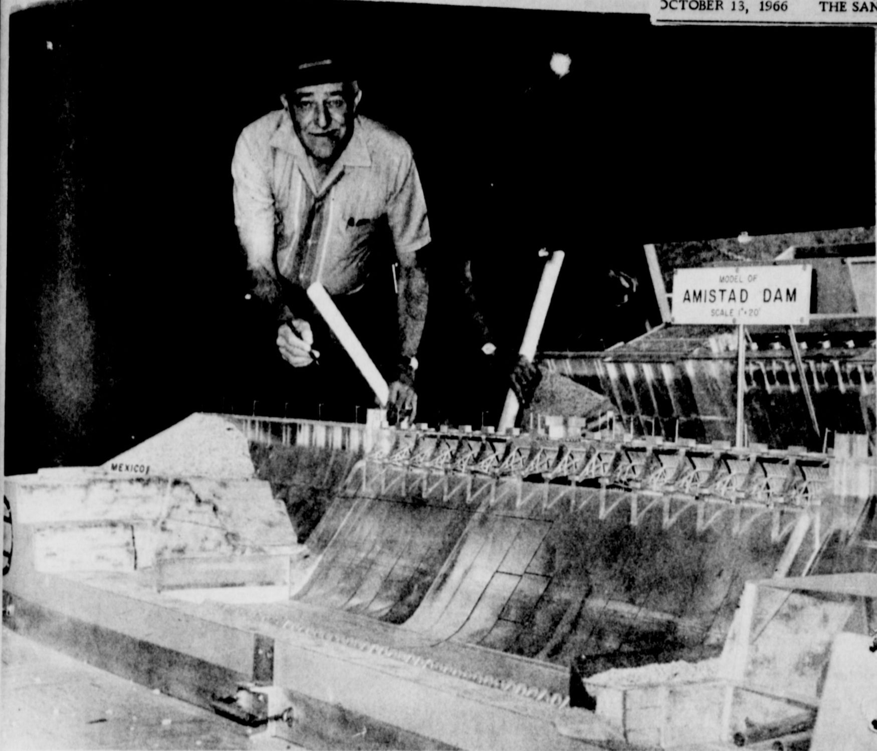
INTERNATIONAL PROJECT—Engineer L. H. Henderson points out features on scale model of Amistad Dam under construction across the Rio Grande in cooperation with Mexico. When completed, the six-mile dam will impound water covering up to 88,200 acres. It will cost about $78 million with completion in late 1968.
