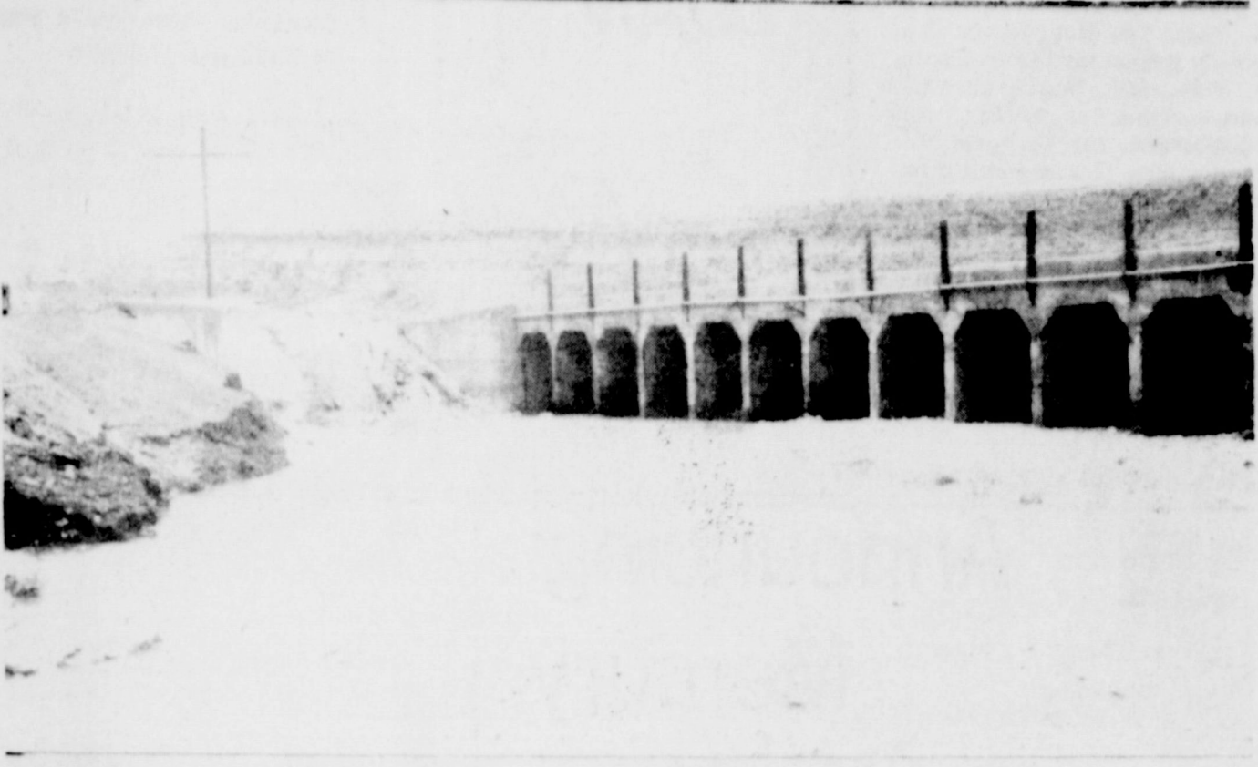
Pictured above is a scene on Sanderson Canyon Friday afternoon of last week following the rain that morning. The water can be seen flowing into the fill that was made following the flood of June 11— and then making the sharp curve to the south - or the right - to negotiate the flumes of the railroad bridge over the canyon bed. The damage to the fill from this small amount of water can be seen on the left. The dirt fill between the east end - or left - of the bridge and the rip-rap which is on the right of the road coming into the canyon can also be seen. --Times photo.
