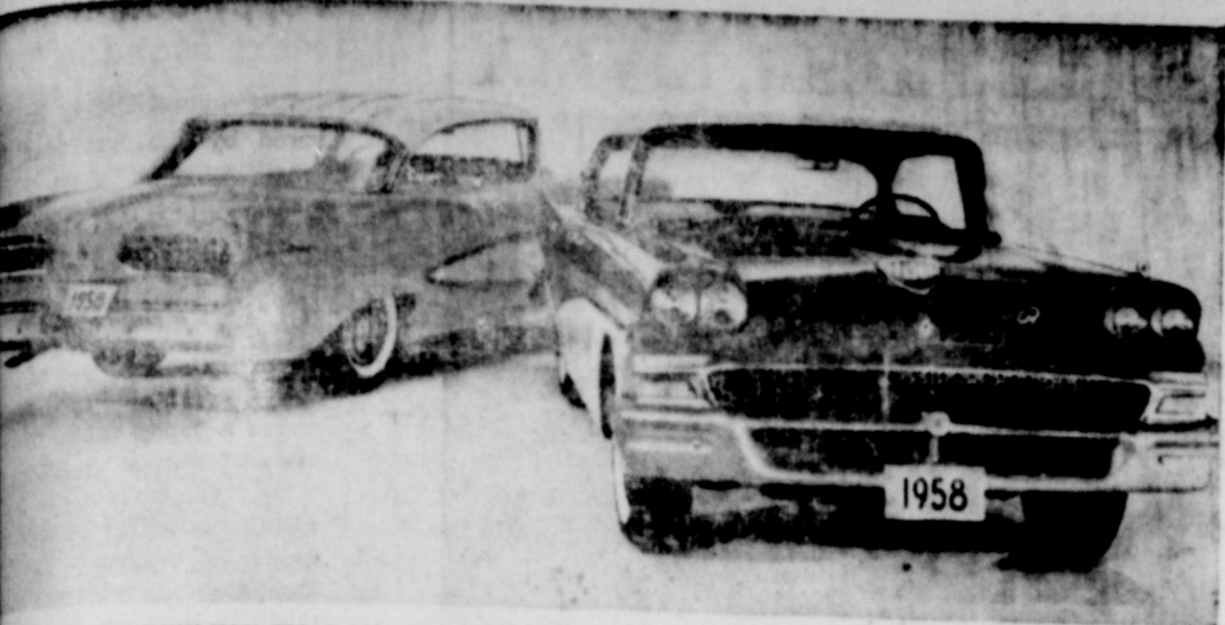
SWEEEPING STYLING CHANGES ARE APPARENT IN THE 1958 FORD CAR LINE. The Fairlane 500 (right) and Fairlane Club Victoria (left) share with all new Fords such dramatic styling changes as new dual headlights, corrosion-proof anodized aluminum grille, power flow hood, slip stream roof, sculptured V-trunk lid and twin safety taillights. Engineering and design advances include new engines, new Cruise-Matic transmission and optional Ford-Aire suspension. The new Ford car line will be on display at Ford dealers on November 7.
