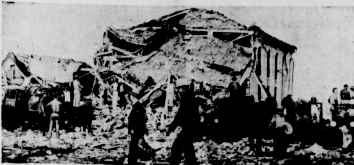
Amid crumbling masonry and steel, rescue workers and frantic parents hunt for bodies of children killed and mangled by explosion.
