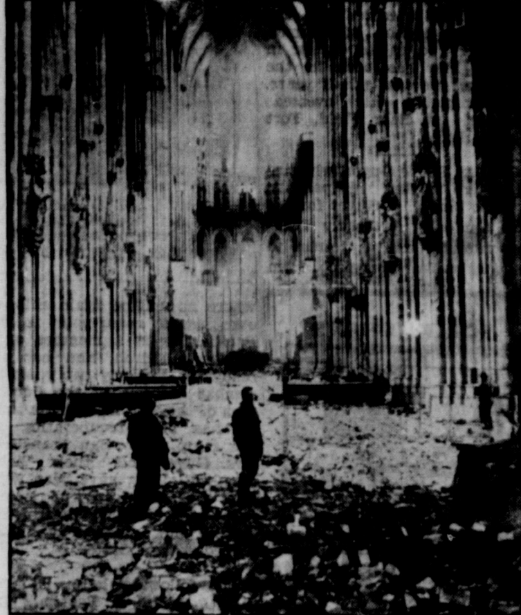
American soldiers survey damage in famed Cologne Cathedral—a litter of masonry from upper regions of the edifice. The Gothic pillars appear undamaged.
