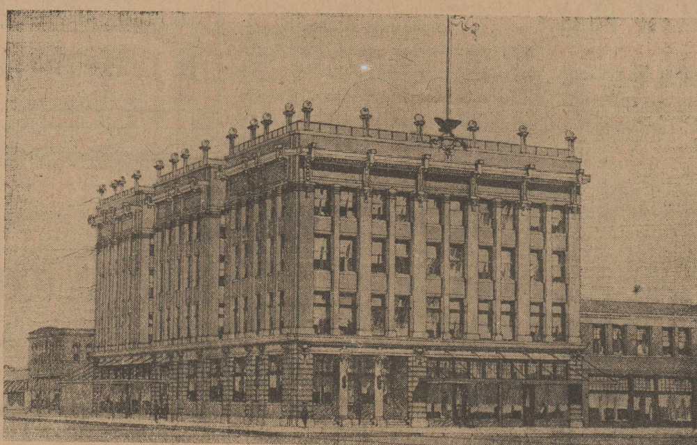
New Midland National Bank and Hotel Building, now under construction at a cost of about $80,000
