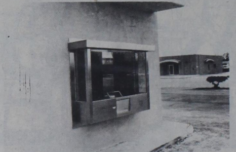
Drive-Up Window on North Side
