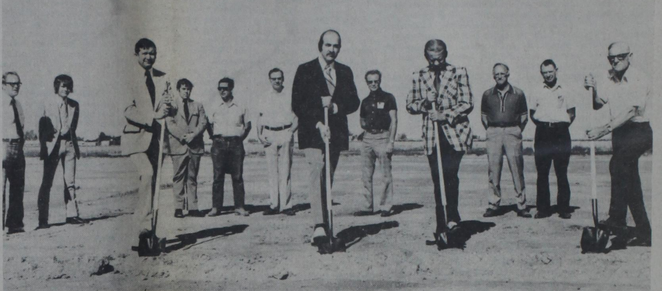
GROUND BREAKING ceremonies for Dale Fowler Ford, Inc., were conducted Monday morning by officials of the Chamber of Commerce and the city as part of a new "growth recognition" program. Turning the first shovels of dirt at the building site on US 385 North are [foreground, from left] Bob Caddell, Chamber of Commerce president; Tom McClure of Accent Building Systems, Inc., of Amarillo, building contractor; Dale Fowler, owner-manager of the local Ford dealership; and Mayor Elmer Youts. Lending moral support in background are [from left] Chamber of Commerce Directors Jerry Marvin, Robert McLean, Jack Edwards, Dan Nelson and Walt Hansen; Bob Baker of Killingsworth Construction Co., concrete contractor; City Commissioner Chet Braafladt, and City Manager-designate Garnett Holland. This was the first such ground-breaking in a new Chamber of Commerce program for new businesses, new construction and expansions. "Our ground-breaking program is intended to publicly recognize those who add to the growth of our city and invest in our future," Caddell explained. "It's very important that the people with this type of faith in our city be recognized."
