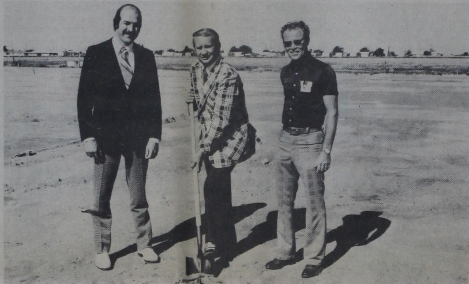
DALE FOWLER turns the first shovel of dirt Monday morning for the new Dale Fowler Ford, Inc., building on US 385 north. With him are representatives of the project's two main contractors — Tom McClure (left) of
