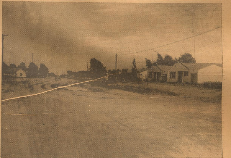
CHANGE COMING —Only one major road in Dimmitt remains unpaved today, but within the next several months it, too, will be hard surfaced. This will be a Farm-to-Market road in North Dimmitt and will be the only east-west paved street in that part of town. It will be paved from its juncture with State Highway 51 at Kirkpatrick Sales Company's location to 25-mile-avenue some six miles west of Dimmitt.
