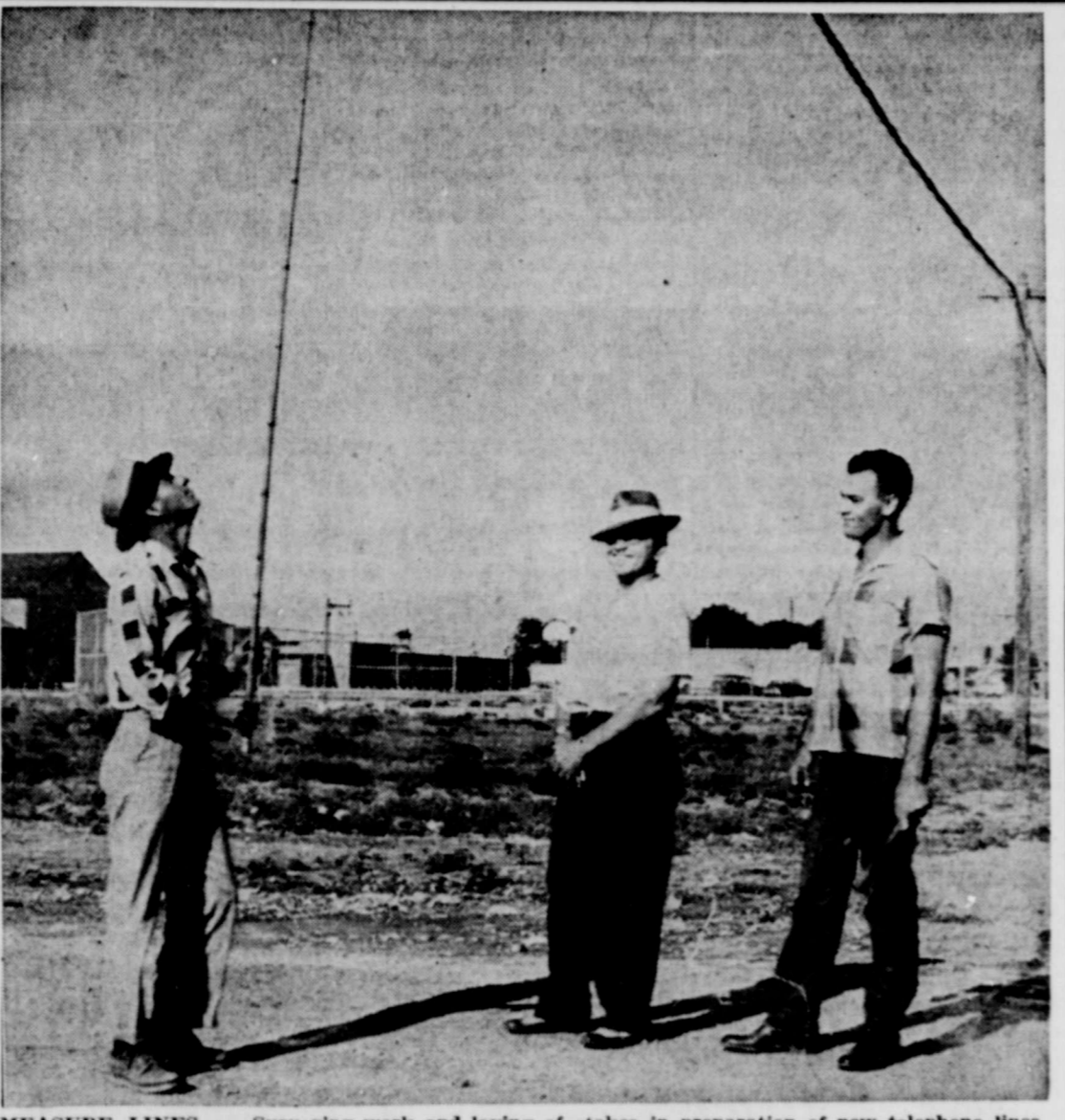
MEASURE LINES — Surveying work and laying of stakes in preparation of new telephone lines began this week in Plains for a new telephone system valued at $300,000 when completed. Pete St. Romain, owner of the local system, confers with G. W. French, left, and Pete Gibson on the changes necessary to existing poles and lines. French and Gibson are employed by Cecil M. Hawk, engineers of Lubbock, contractors for the job. REVIEW Photo
