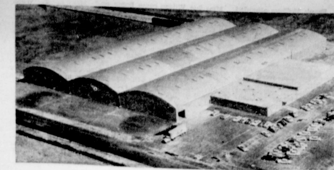
IT HAD TO BE an aerial photo to show the vast size of the new Affiliated Food Store Warehouse at 6700 S. Washington, Amarillo. Offices of the organization and vaults for frozen foods and cheese are housed in the masonry portion at the right, while the receiving and shipping docks and the rail car docks are in the steel building. Sixteen trucks deliver merchandise from the big warehouse to Affiliated Stores of the tri-state area.
