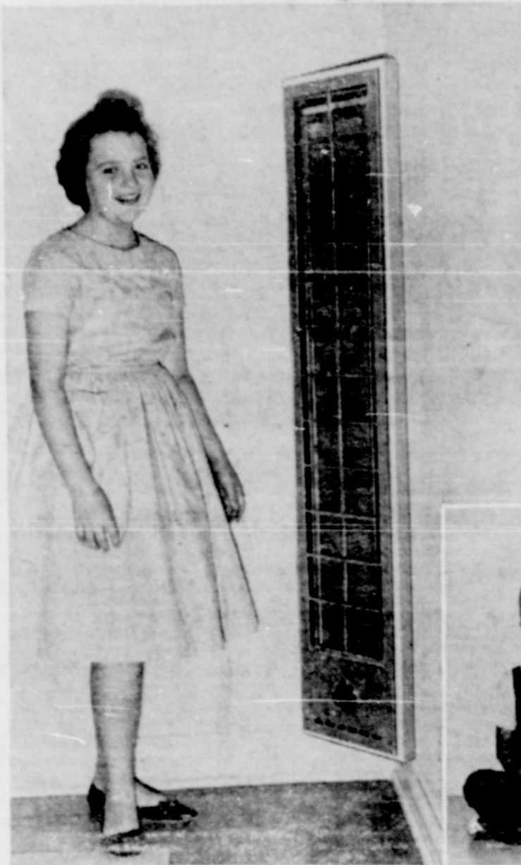
"Independent room control" is feature of electric heating system at H. H. Miller farm, Dawn, Texas. Radiant glass panels make attractive and safe installation and give exact degree of heating desired.
